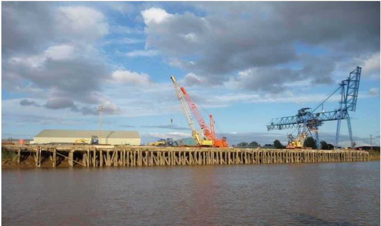
Figure 2-6 - Photograph of Flixborough Wharf (source: [REDACTED])
